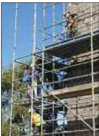
Work nearing completion at St Audoen's.
